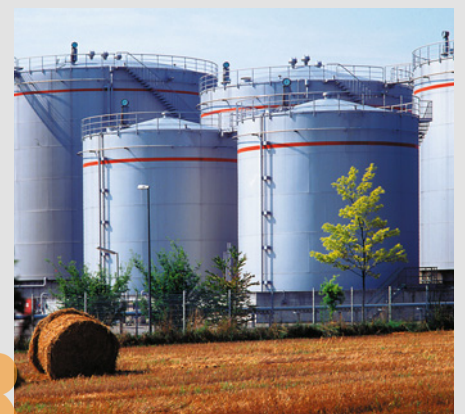
Industrial steel constructions
